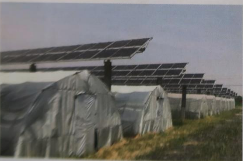
Figure 36: PV modules cover a foil tunnel.
