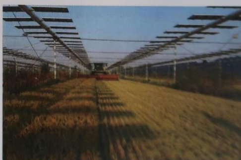
Figure 30: System with high mounting structure and selective function in the Netherlands. © BayWa r.e.
