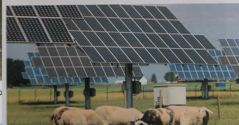
Figure 30: System with high mounting structure and selective function in the Netherlands. © BayWa r.e.
