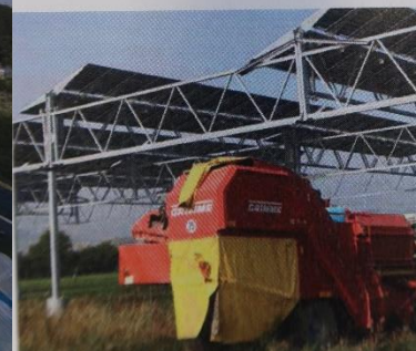
Figure 30: System with high mounting structure and selective function in the Netherlands. © BayWa r.e.
