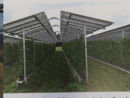
Figure 30: System with high mounting structure and selective function in the Netherlands. © BayWa r.e.
