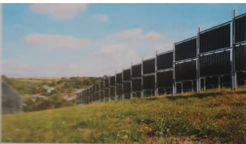
Figure 35: Bifacial modules installed vertically, Donaueschingen. © Next2Sun GmbH
